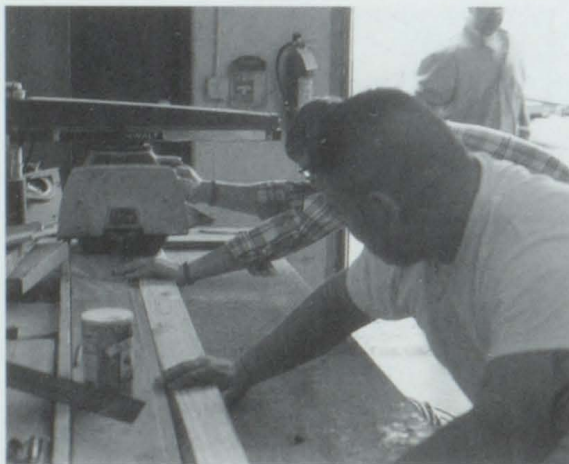
Above: Austin and CJ work together to cut a 2x4.
