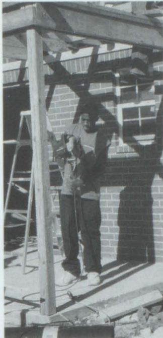
Kenneth framing a storage building.
