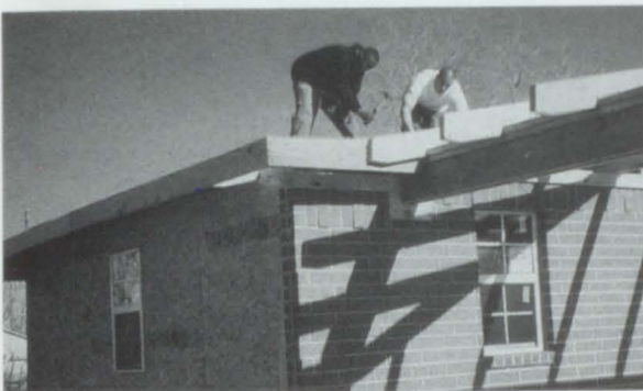
Above: Kevin and Jeremiah installing decking on the roof.
