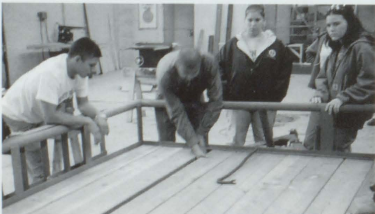
Albert, Jose Medina, Laura Vesper, and Kelly Clardy placing boards on the VFW trailer.
