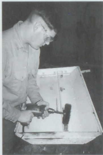
MATT HUEBNER BUFFING RUST OFF OF A LIGHT FIXTURE.
