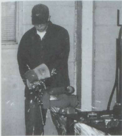
MATT MOTE GRINDING PIPE FOR A PROJECT.
