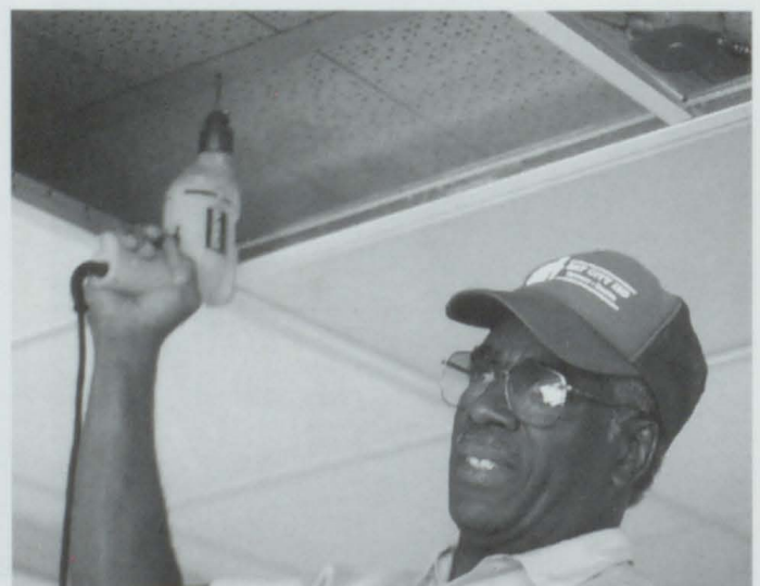
MR. WIGGINS FIXING THE LIGHTING IN THE CEILING.
