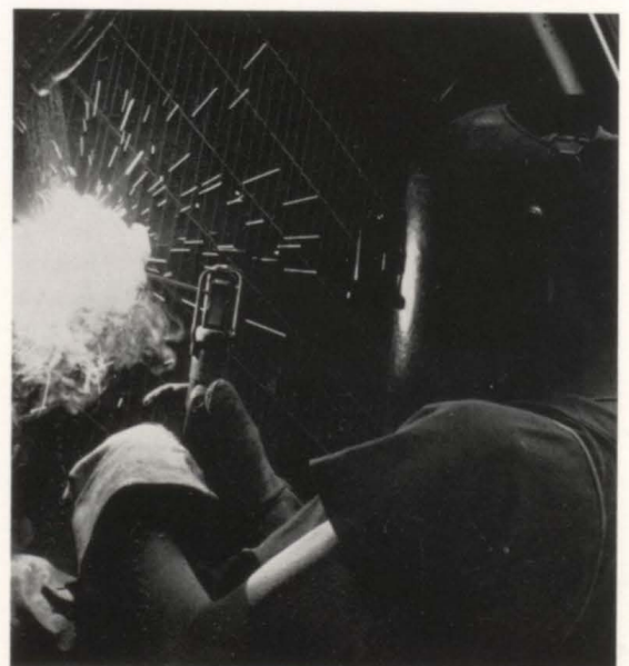
ELECTRIC WELDING Jerry Castleberry working on a project.
