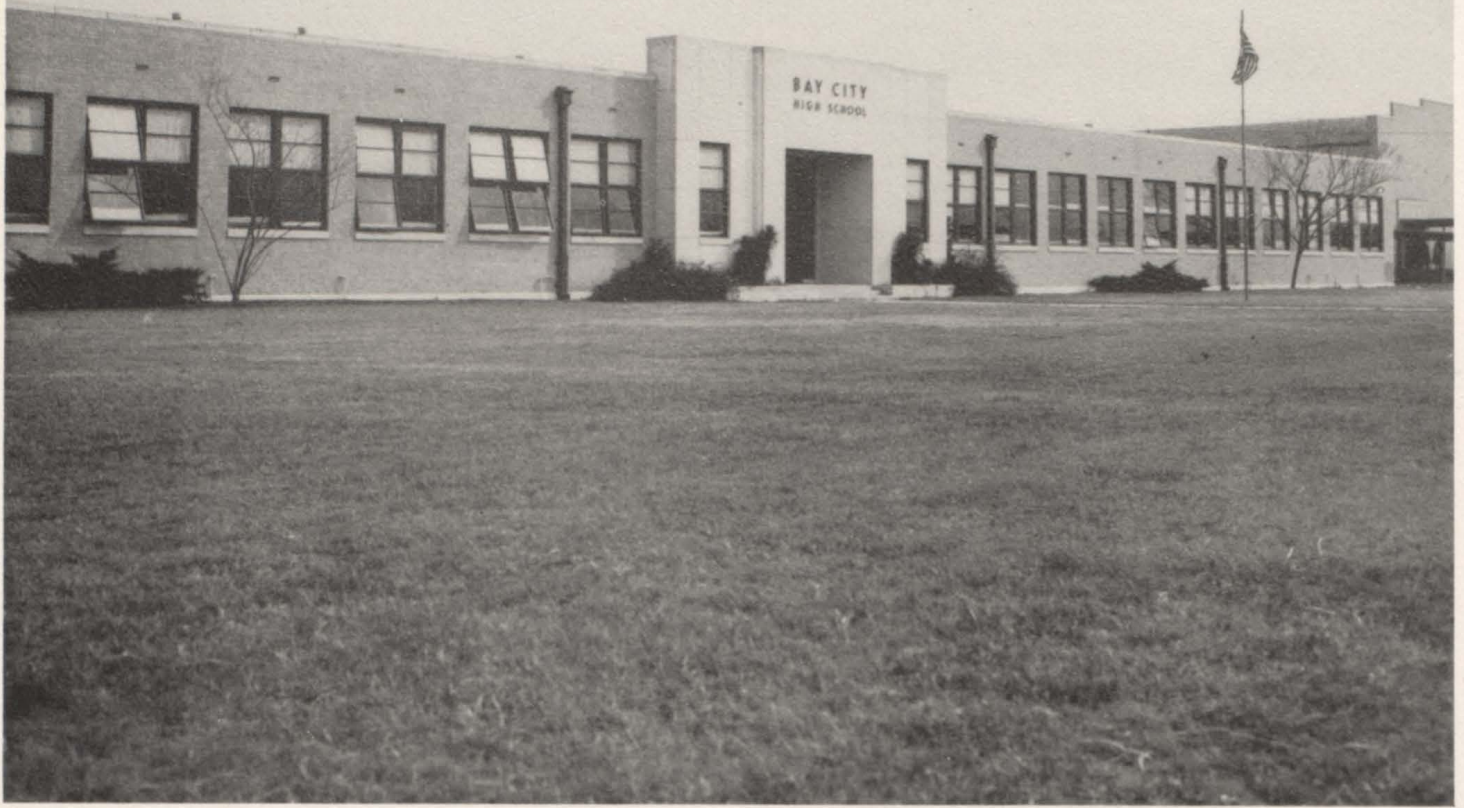
MAIN BUILDING BAY CITY HIGH SCHOOL
