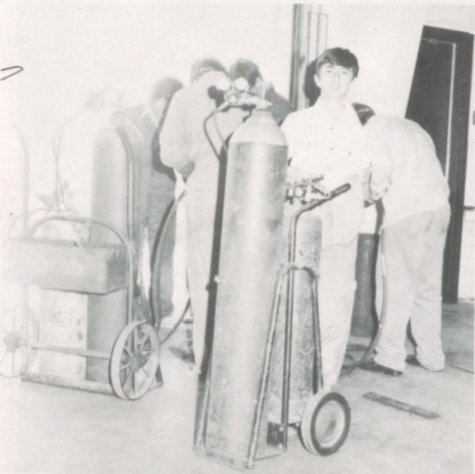
VA I Students practicing acetylene cutting.
