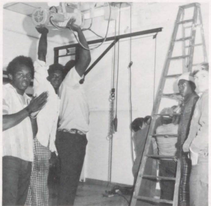
Students installing backsaw in kill room.
