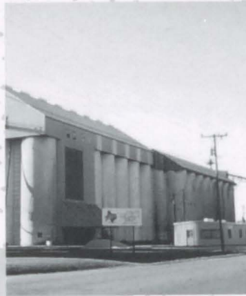
Rice Belt Warehouse, Blessing
