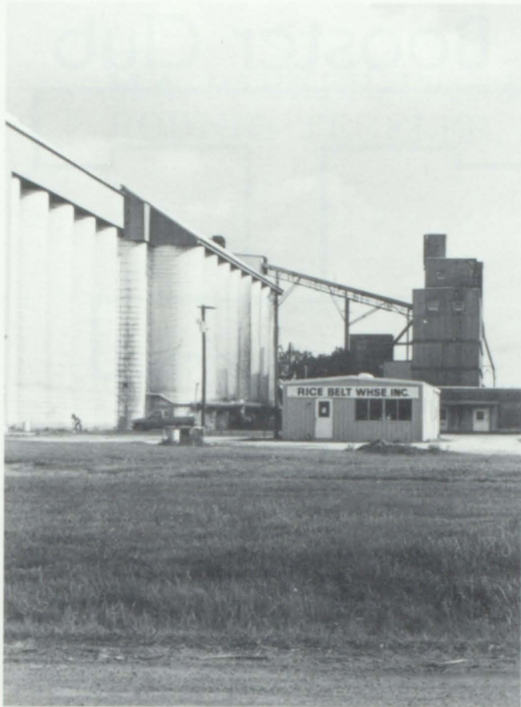
The Rice Belt Warehouse is the major industry of Blessing.
