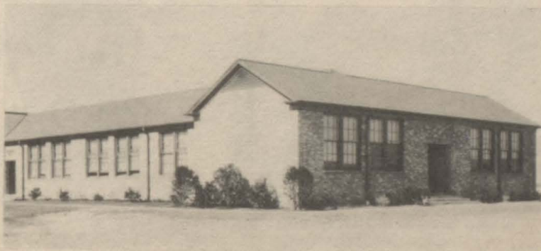
ELEMENTARY SCHOOL BUILDING
